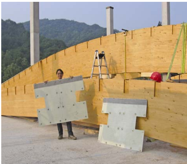
Figure 30: Example of Giunto Italia ® with double GFRP inserts
